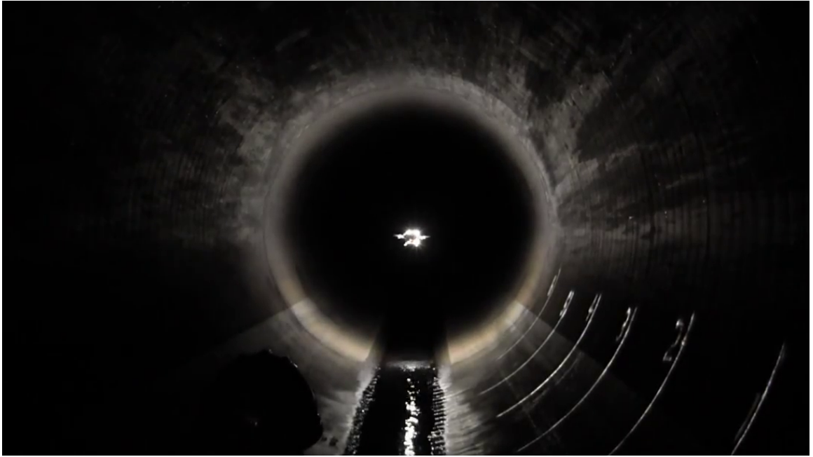
Figure 3.6: A photo taken from inside a penstock at Glen Canyon Dam, AZ while the KHex platform is flying autonomously. The robot is tested for visual odometry with onboard LEDs as the only source of illumination.
