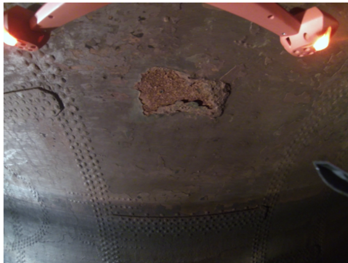
Figure 3.4: An image from inside a penstock in Allatoona Dam, GA. This image was taken from a quadcopter flown manually close to a patch that needs maintenance.
