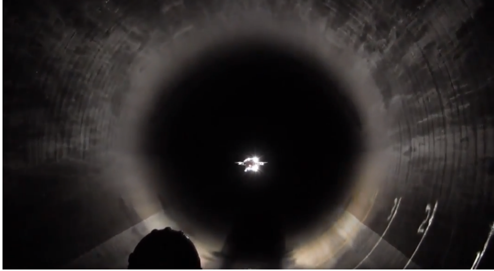
Figure 5.12: A snapshot from the experiments inside a penstock at Glen Canyon Dam, AZ. The robot is flying fully autonomously using onboard illumination. Also, in Fig. 5.11 and Fig. 5.10, we show the local 3D reconstruction and the 360 degrees panoramic image generated using the images from the onboard four cameras.
