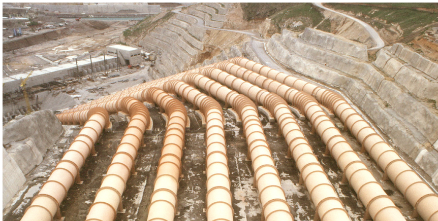
Figure 3.1: An array of steel penstocks.
